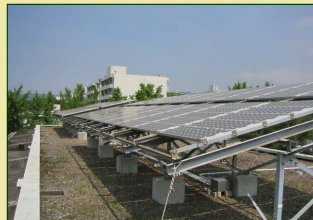
10 kW photovoltaic experimental generation system
